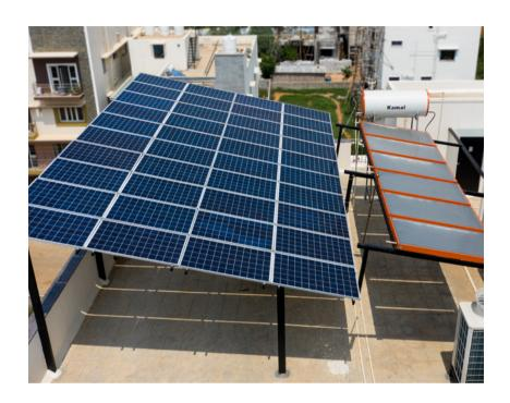
Hybrid system is best suited for places with power, but with frequent power cuts. In case of excess power generated, the power is supplied back to the grid. If the grid is not available (during power cut), the building will still have electrical supply due to the batteries connected to the inverter.
