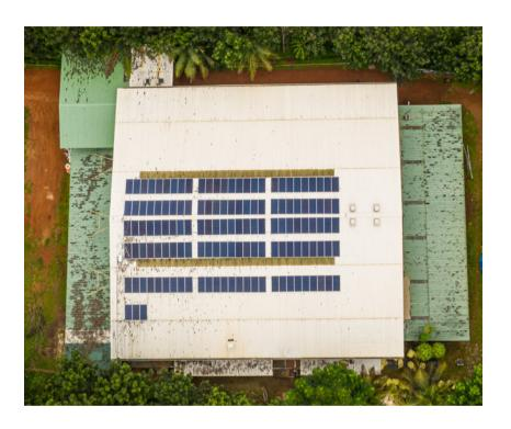
On-Grid Solar Rooftop is best suitable for places with constant power supply. In this case, the excess generated power is supplied back to the grid where the government pays the per unit cost back to the client. This involves permission from the electricity board.
